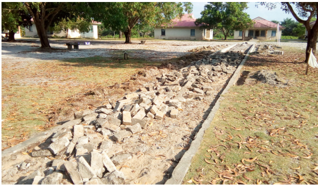
Work on the sidewalks continues
